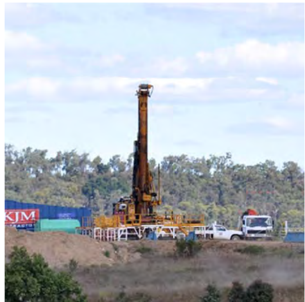
Plate 20-23 Production Well Drilling (Source GBD, 2012)
