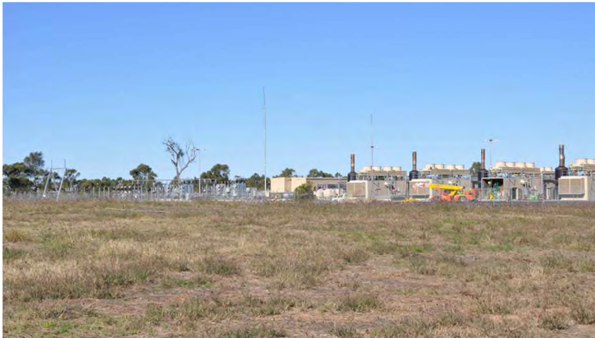
Plate 20-35 Gas Fired Power Plant, Generators and Local Substation (Source GBD, 2012)
