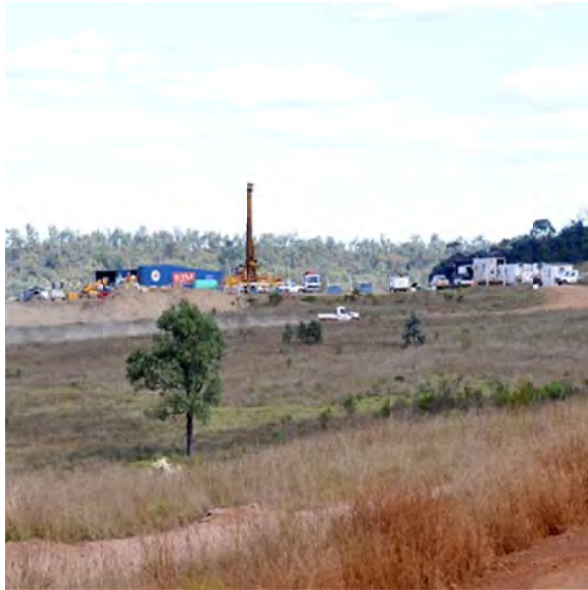
Plate 20-22 Production Well Drilling (Source GBD, 2012)
