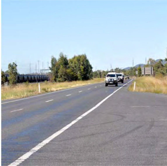
Plate 20-12 Peak Downs Highway (Source GBD, 2012)
