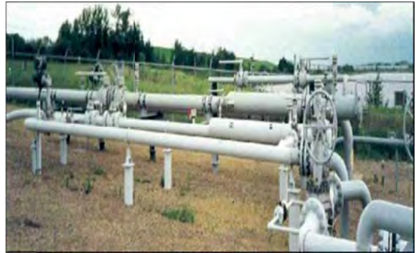
Plate 20-29 Pig Station Launcher (Source Arrow, 2012)
