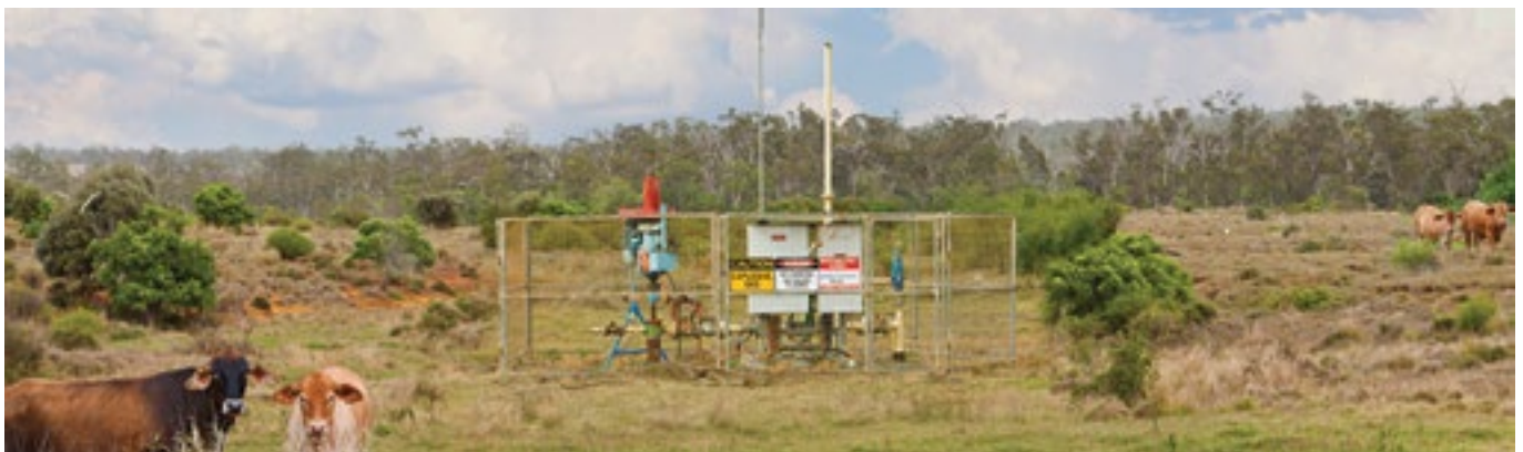
Plate 1. Typical Production Wellhead
