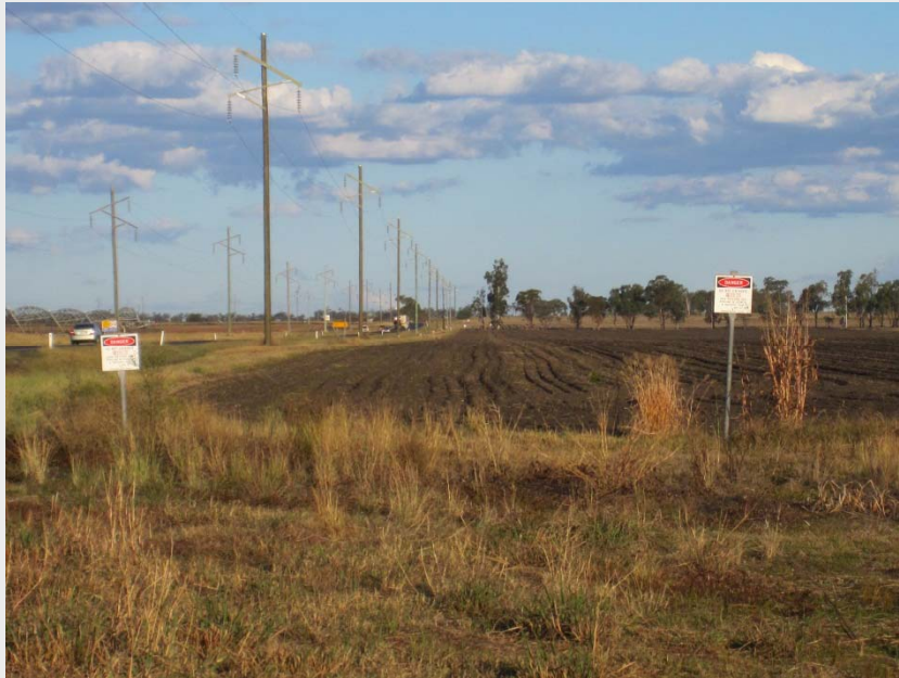
Roma-Brisbane Pipeline – Warrego Highway
