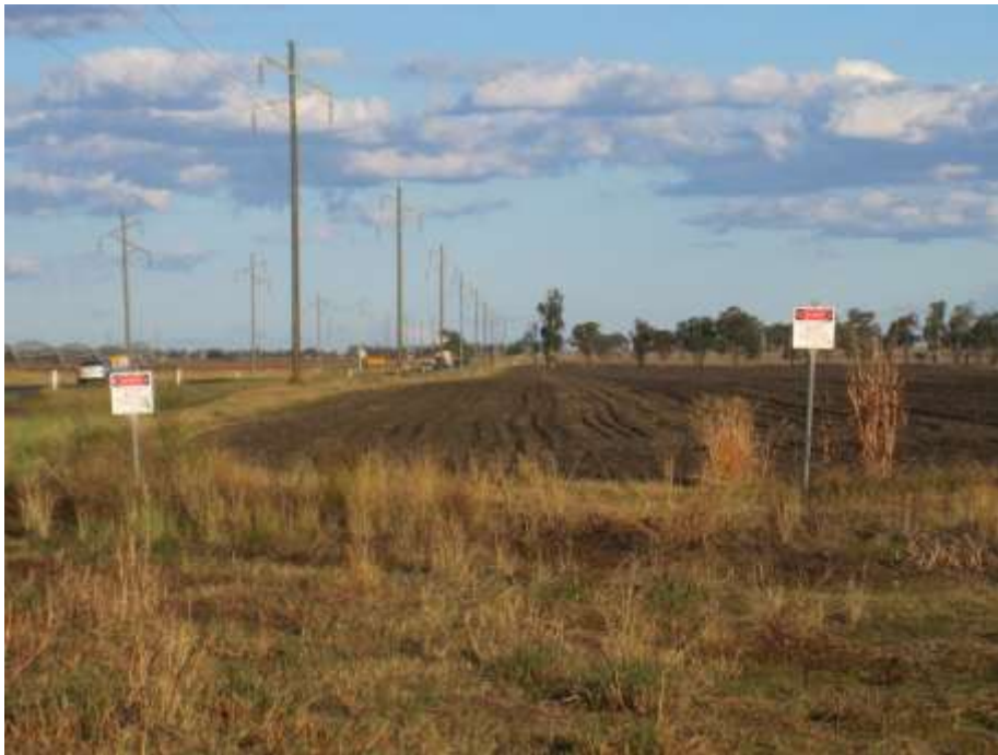
Figure 7 – Roma – Brisbane pipeline, Warrego Highway
