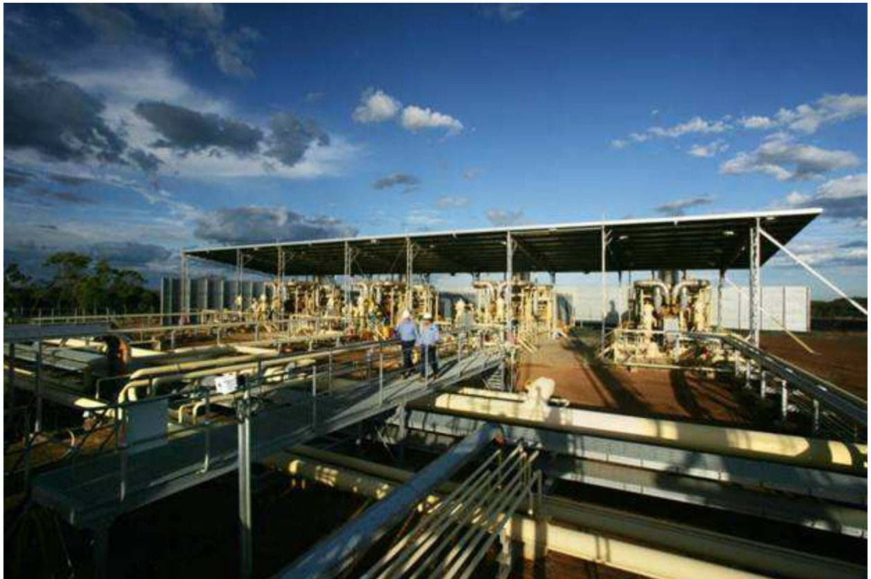
Figure 4 - Moranbah gas processing facility
