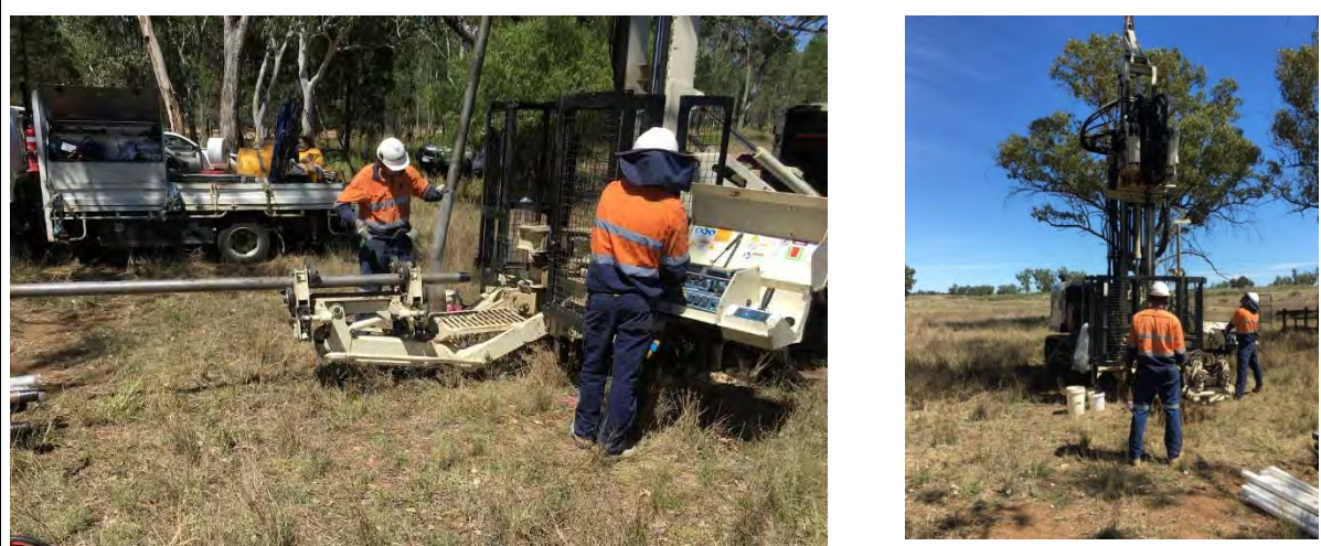
Photograph 18 & 19. Sonic Rig coring and installing monitoring bores on Wambo Ck.
