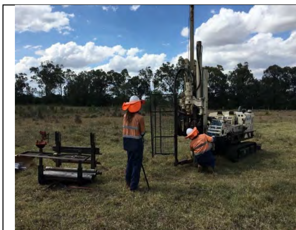
Photograph 16. Geoprobe rig coring and installing monitoring bores on the CRA.
