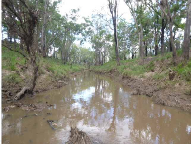
DA2-7 – Dogwood Creek (Looking Upstream)
