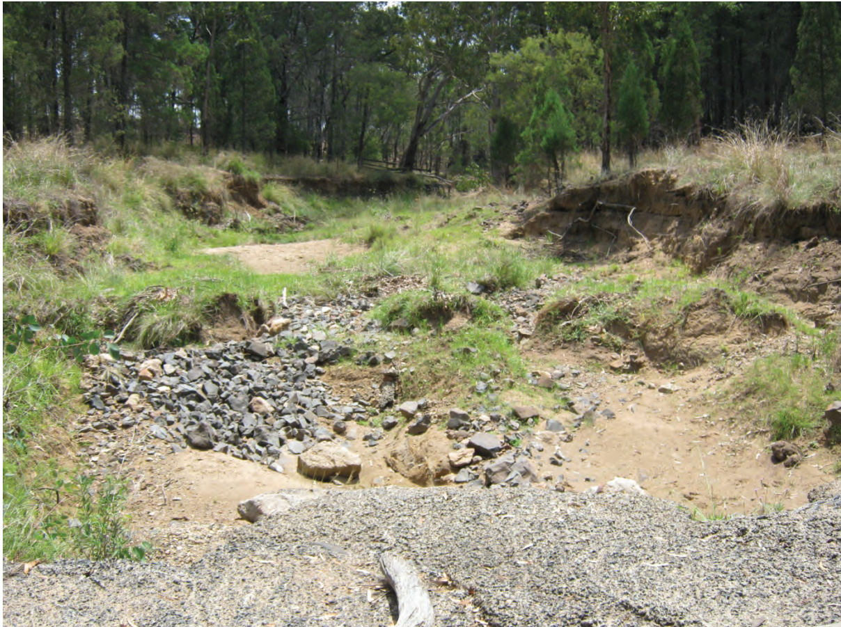
Figure 108: River crossing, view to Southwest
