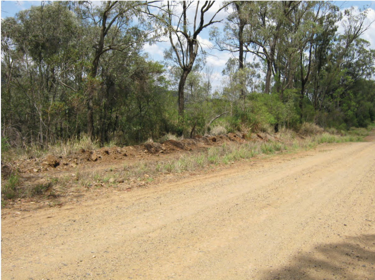
Figure 116: Road cutting, view to East
