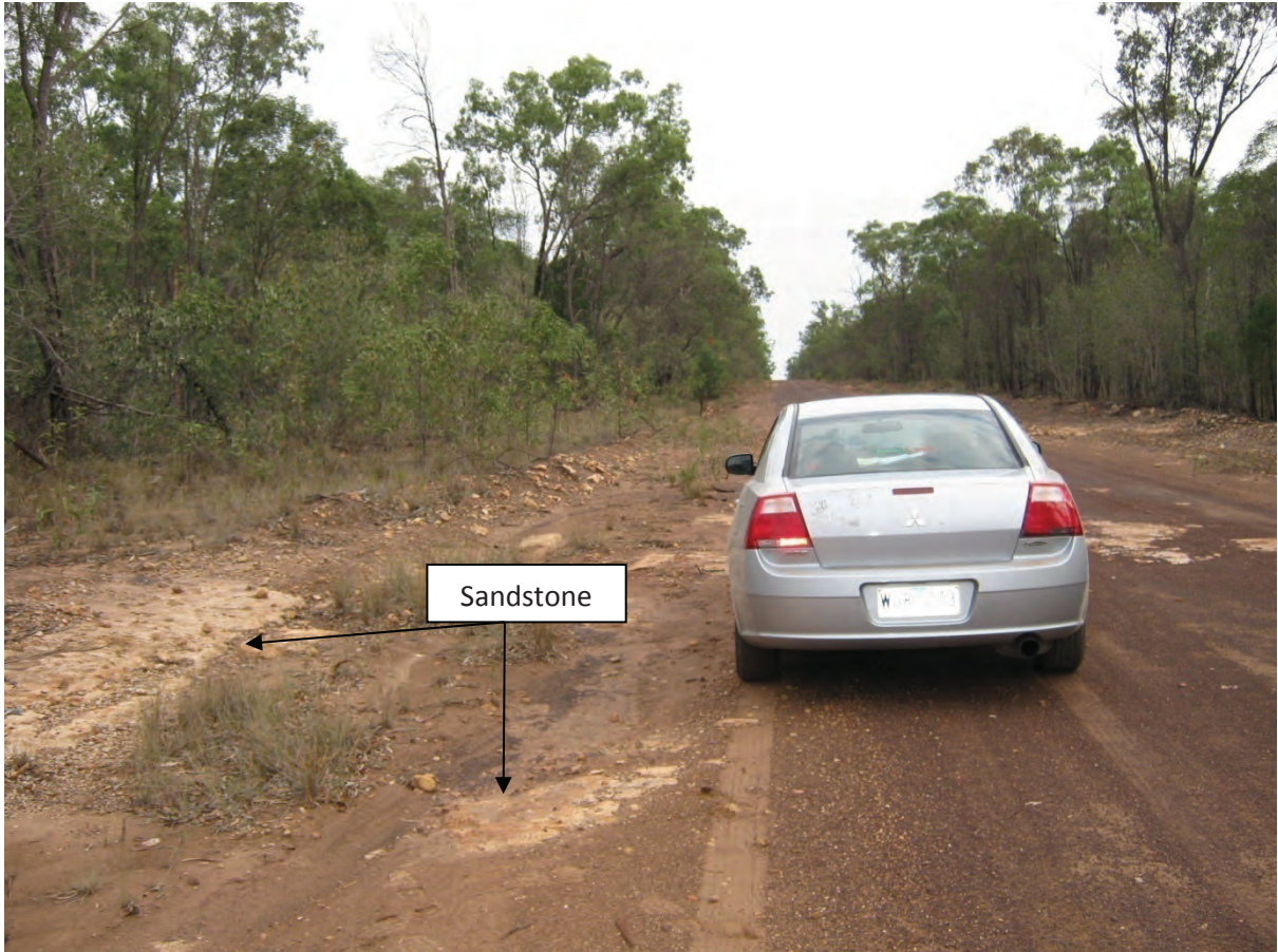
Figure 21: Road drain, view to North
