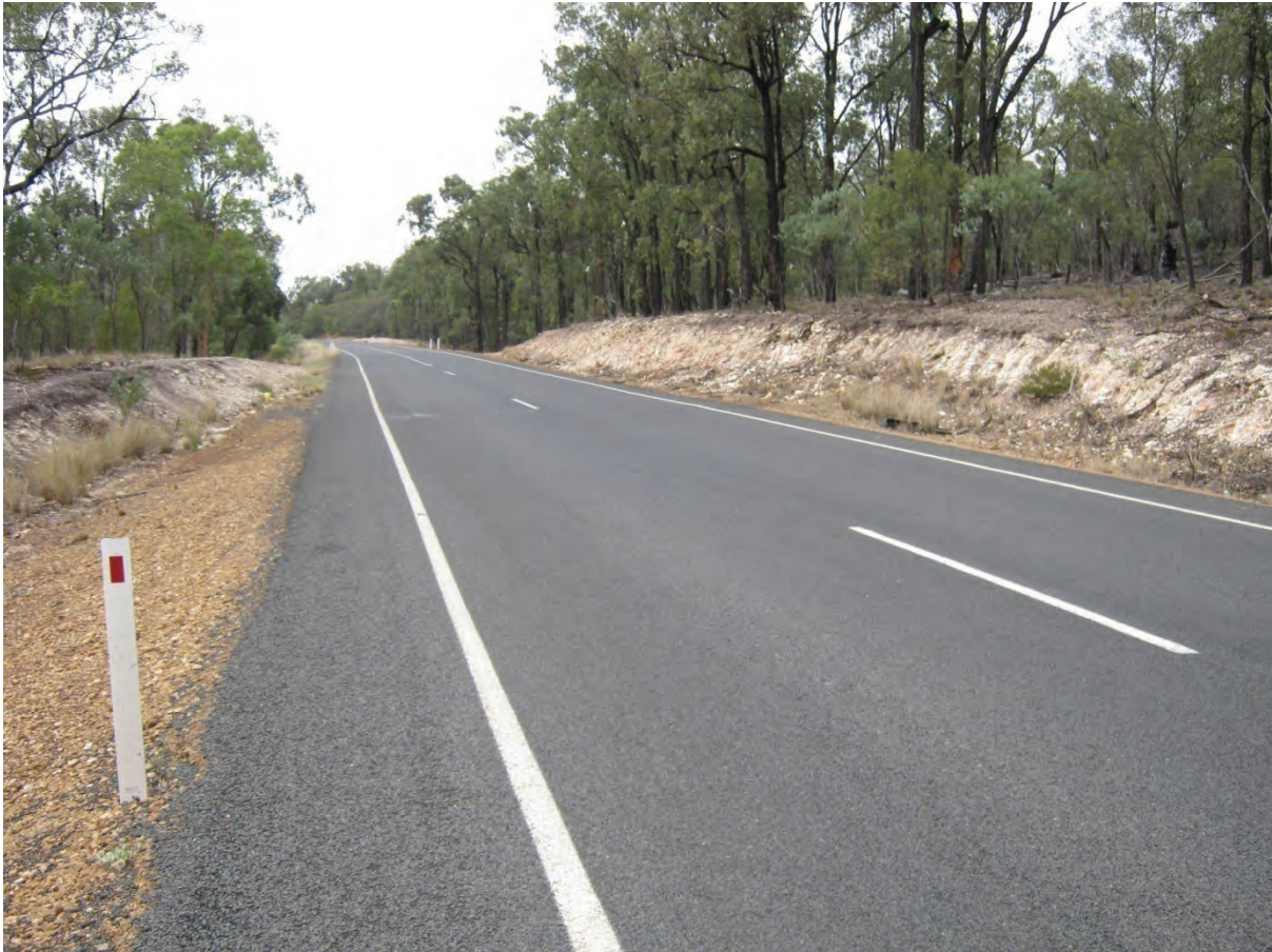
Figure 30: Road cutting, view to South
