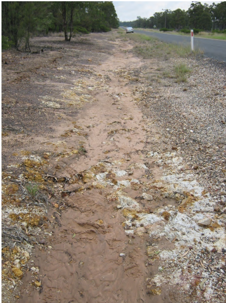
Figure 59: Road drain, view to West - Southwest
