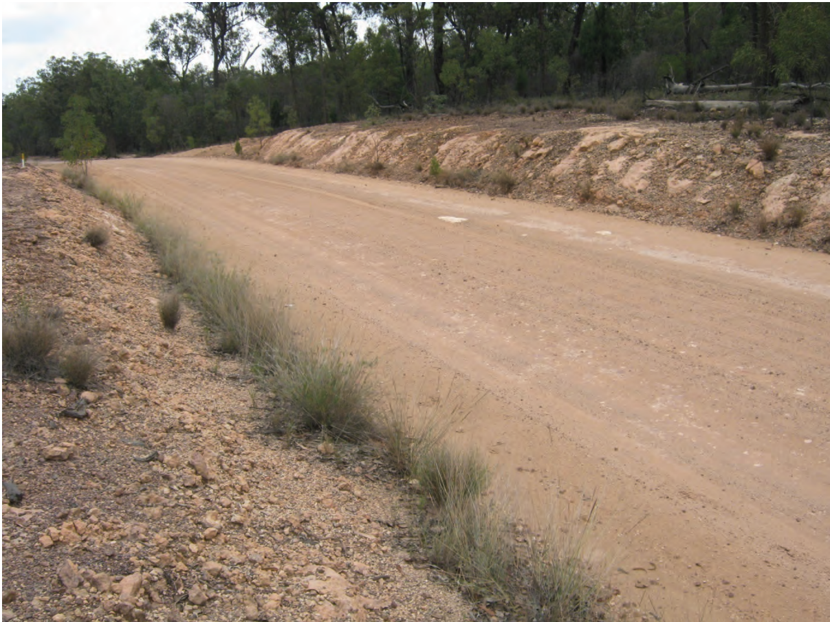
Figure 54: Road cutting, view to West
