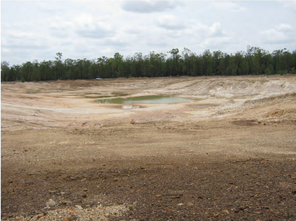
Figure 37: Borrow pit, view to Southeast
