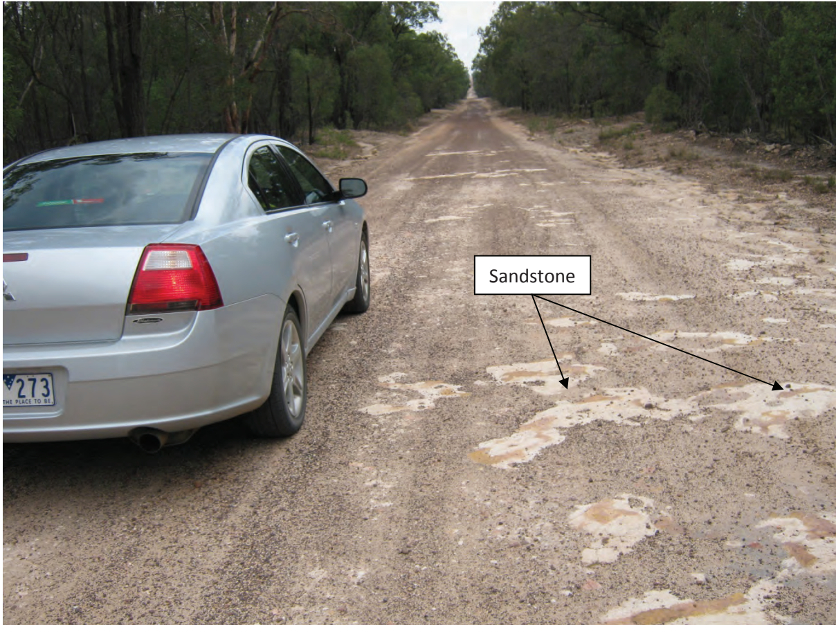
Figure 61: Road, view to South
