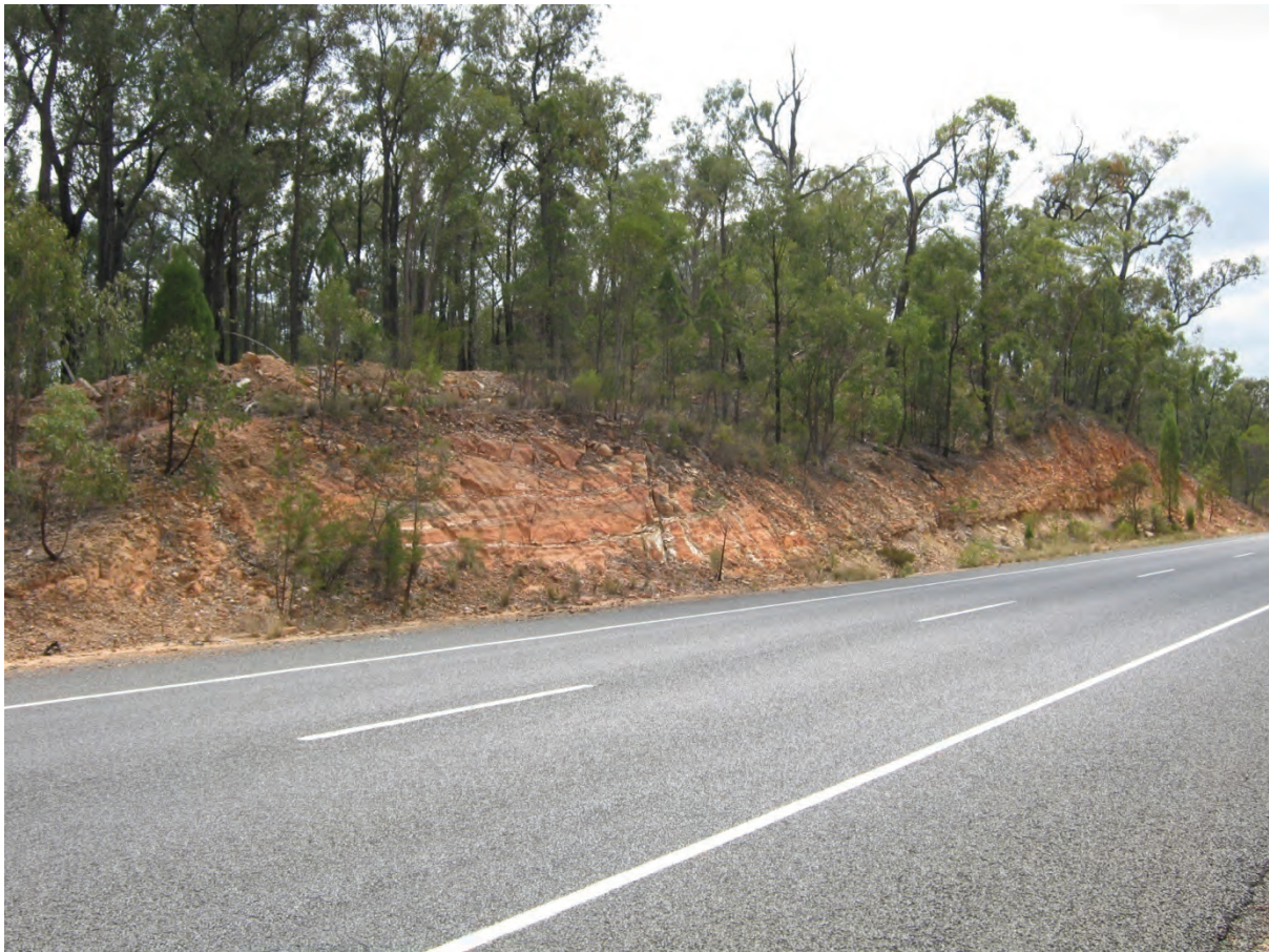
Figure 87: Road cutting, view to Northeast
