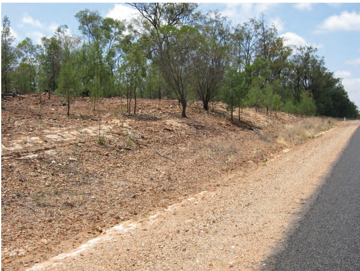
Figure 93: Road cutting, view to Southeast
