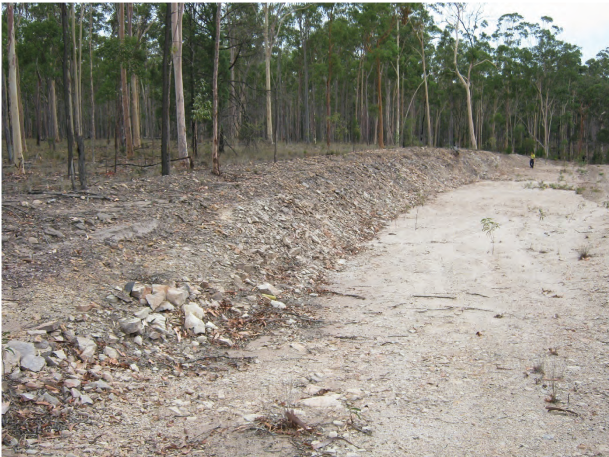
Figure 29: Road cutting, view to East
