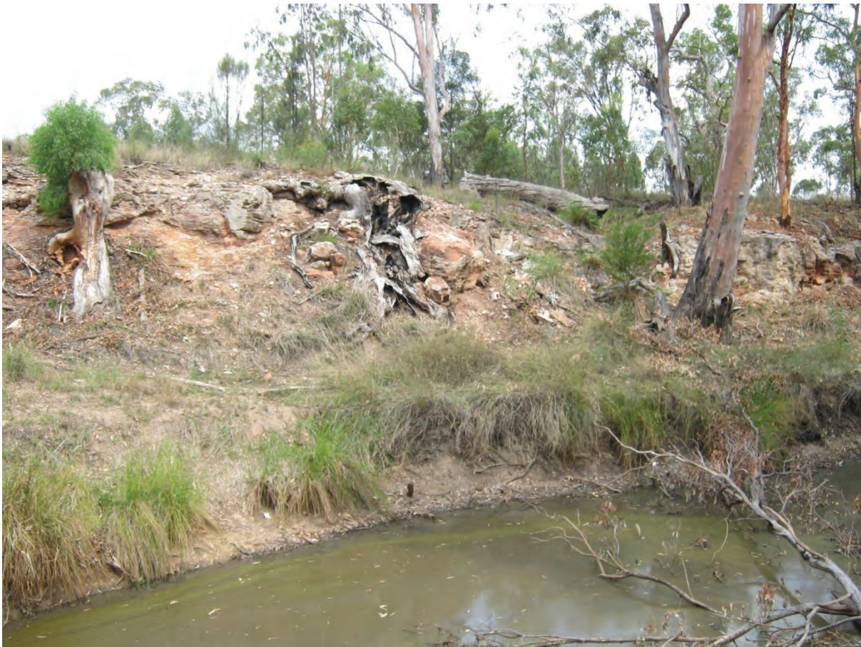
Figure 63: Creek embankment, view to East
