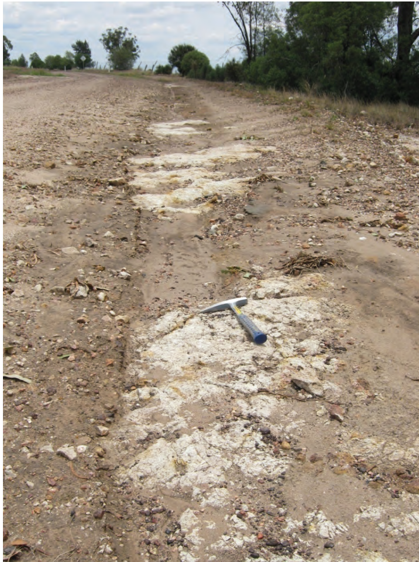
Figure 100: Road drain view to North – Northwest
