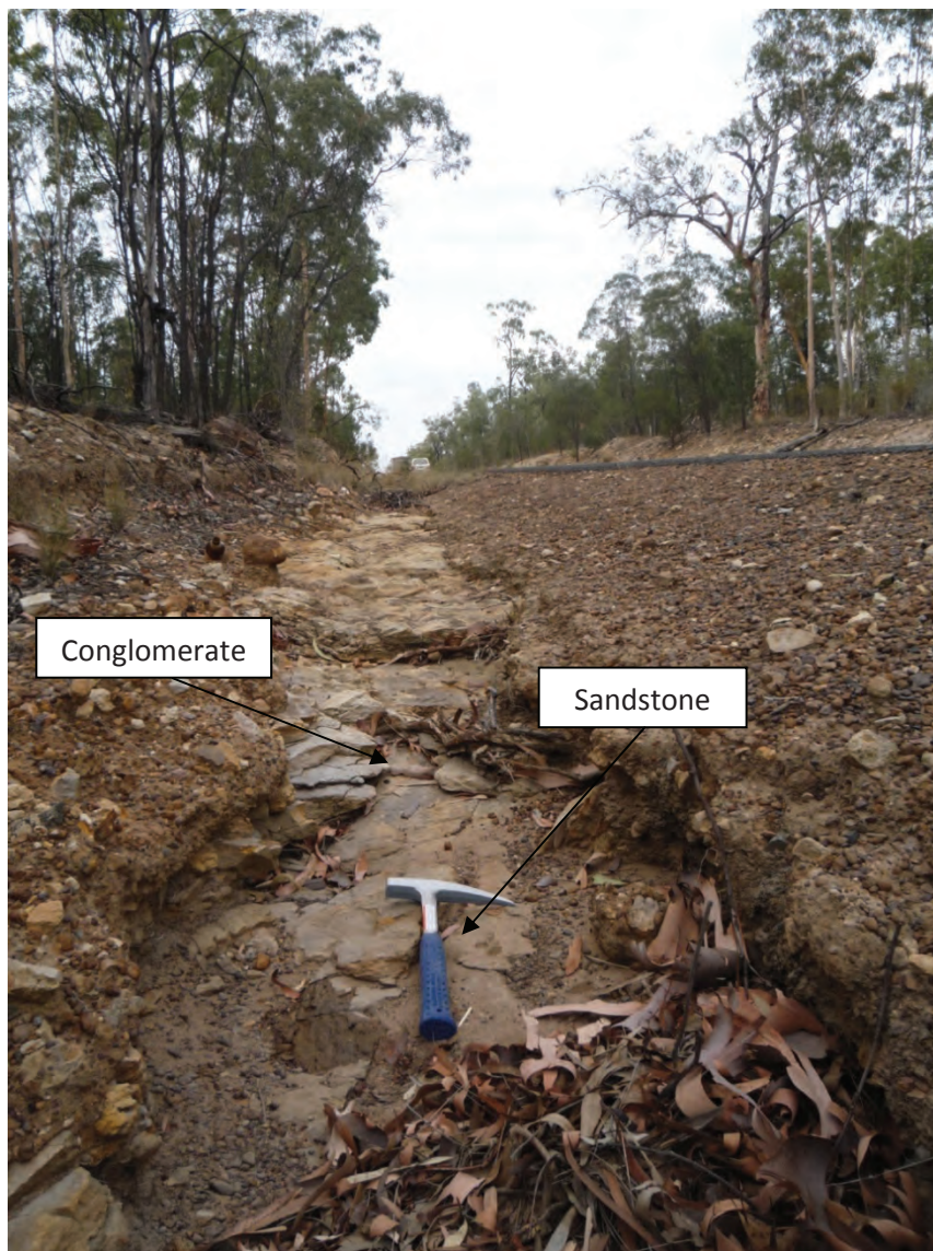
Figure 13: Road cutting and road drain, view to North – Northwest
