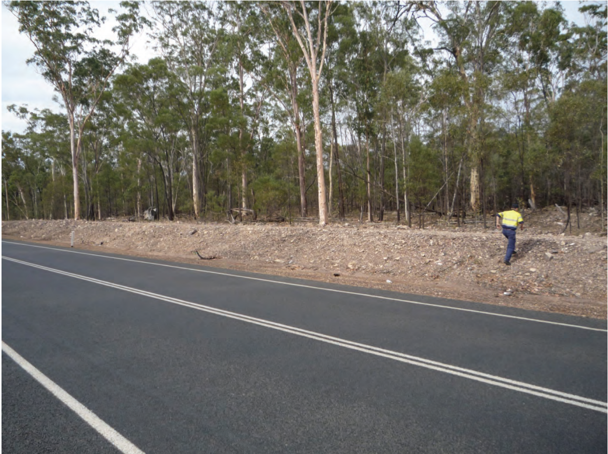
Figure 15: Road cutting, view to North
