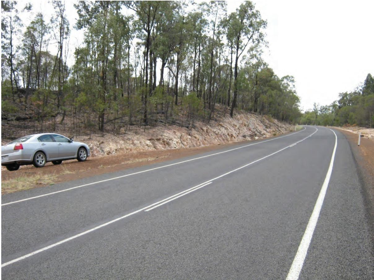
Figure 32: Road cutting, view to Southeast
