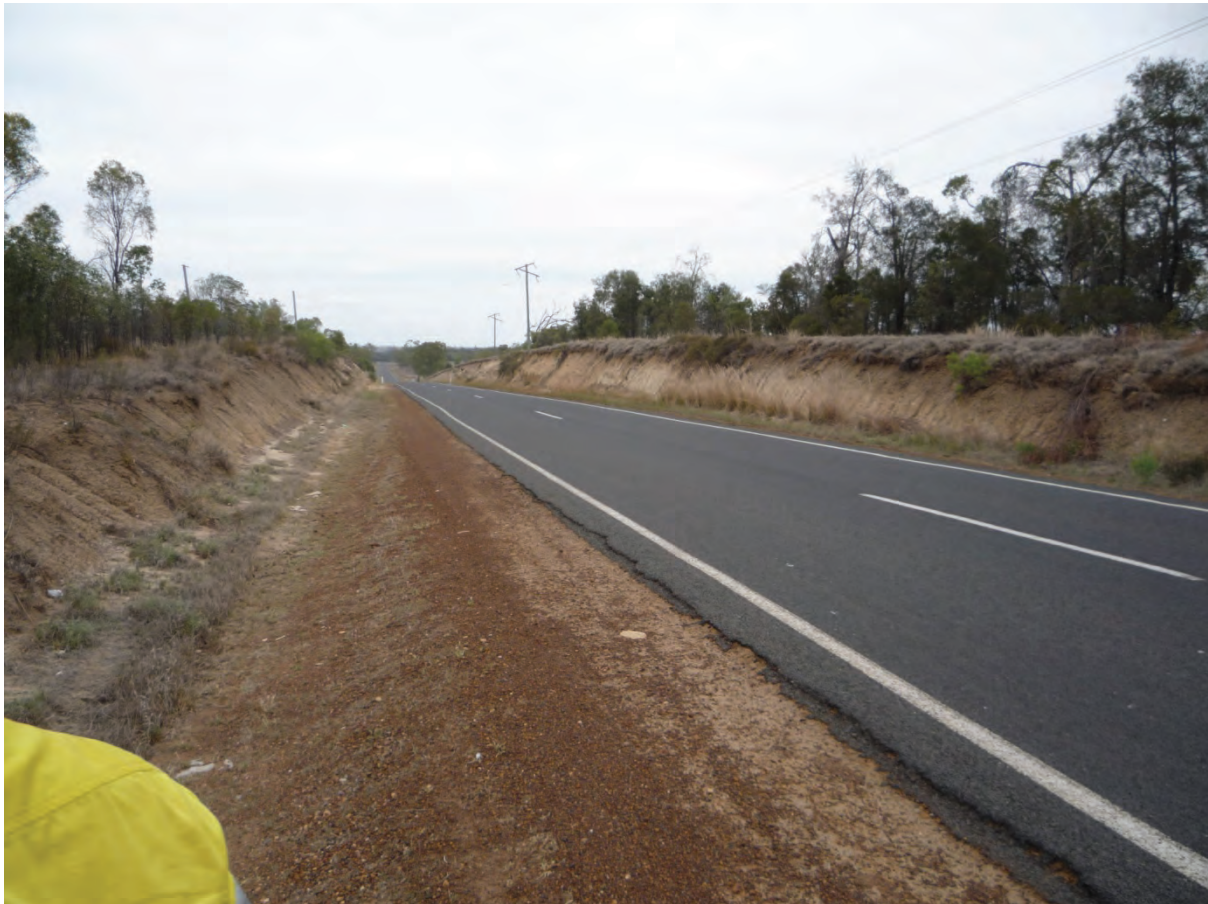
Figure 3: Road cutting, view to South
