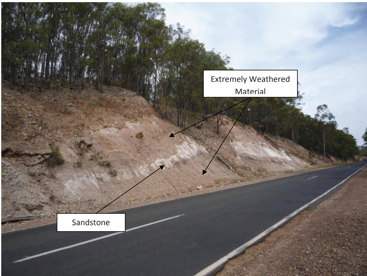
Figure 10: Road cutting, view to Northeast
