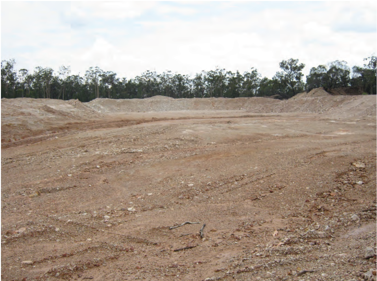
Figure 51: Borrow pit, view to South
