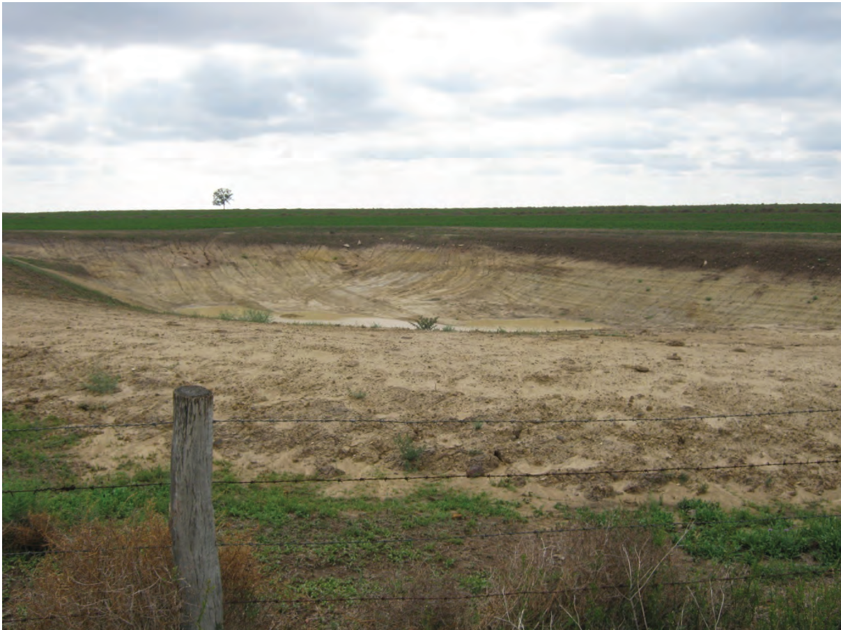
Figure 80: Dam excavation, view to East
