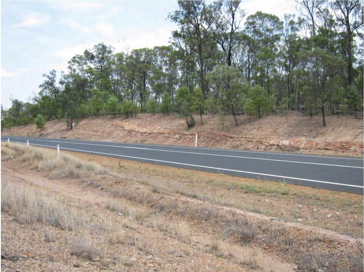
Figure 35: Road cutting, view to North
