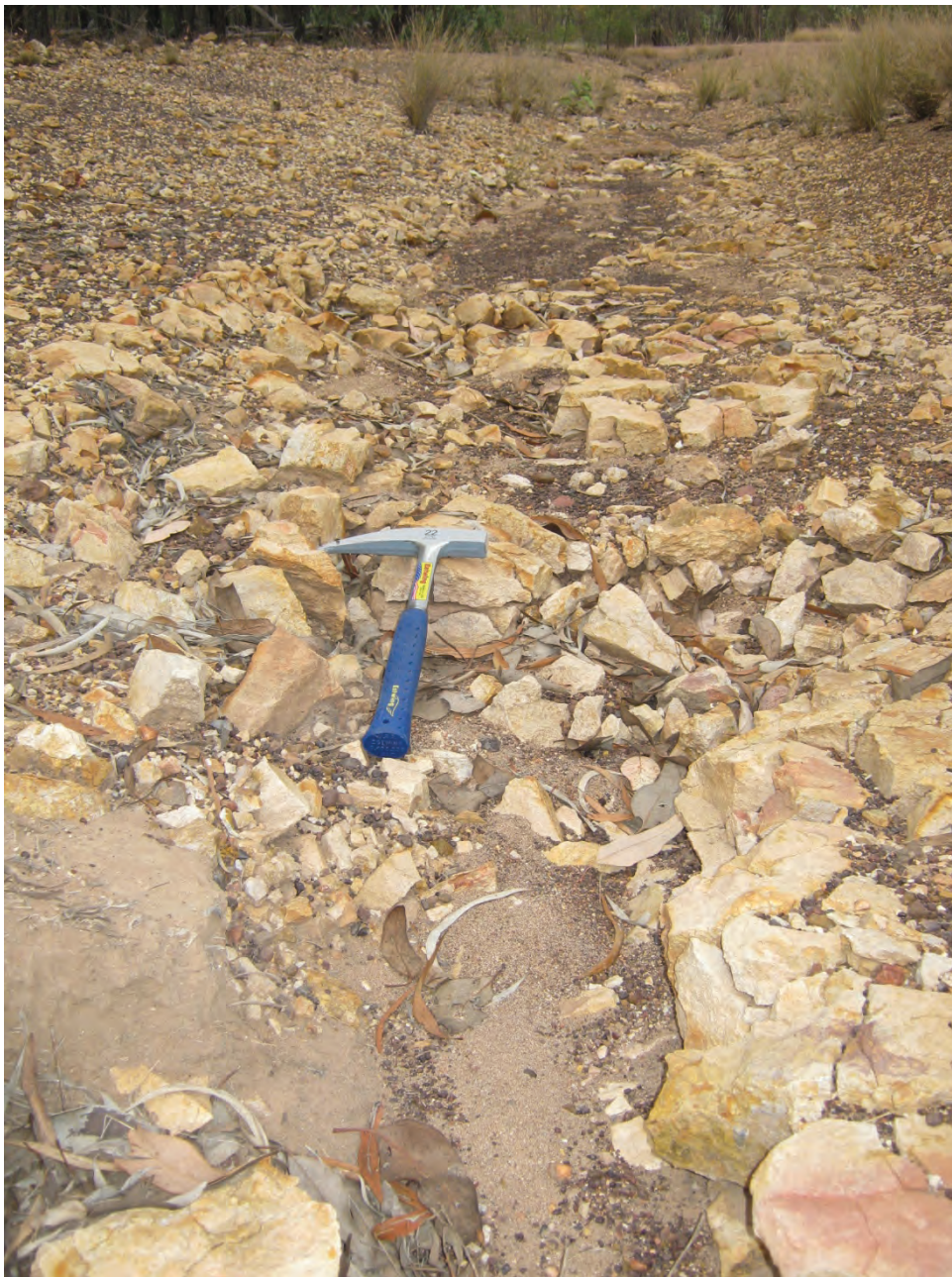
Figure 20: Road drain, view to Southwest
