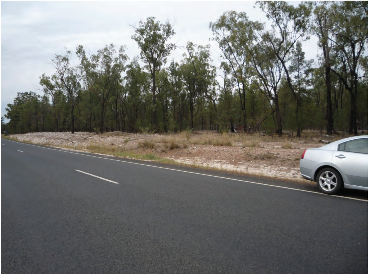
Figure 16: Road cutting, view to North
