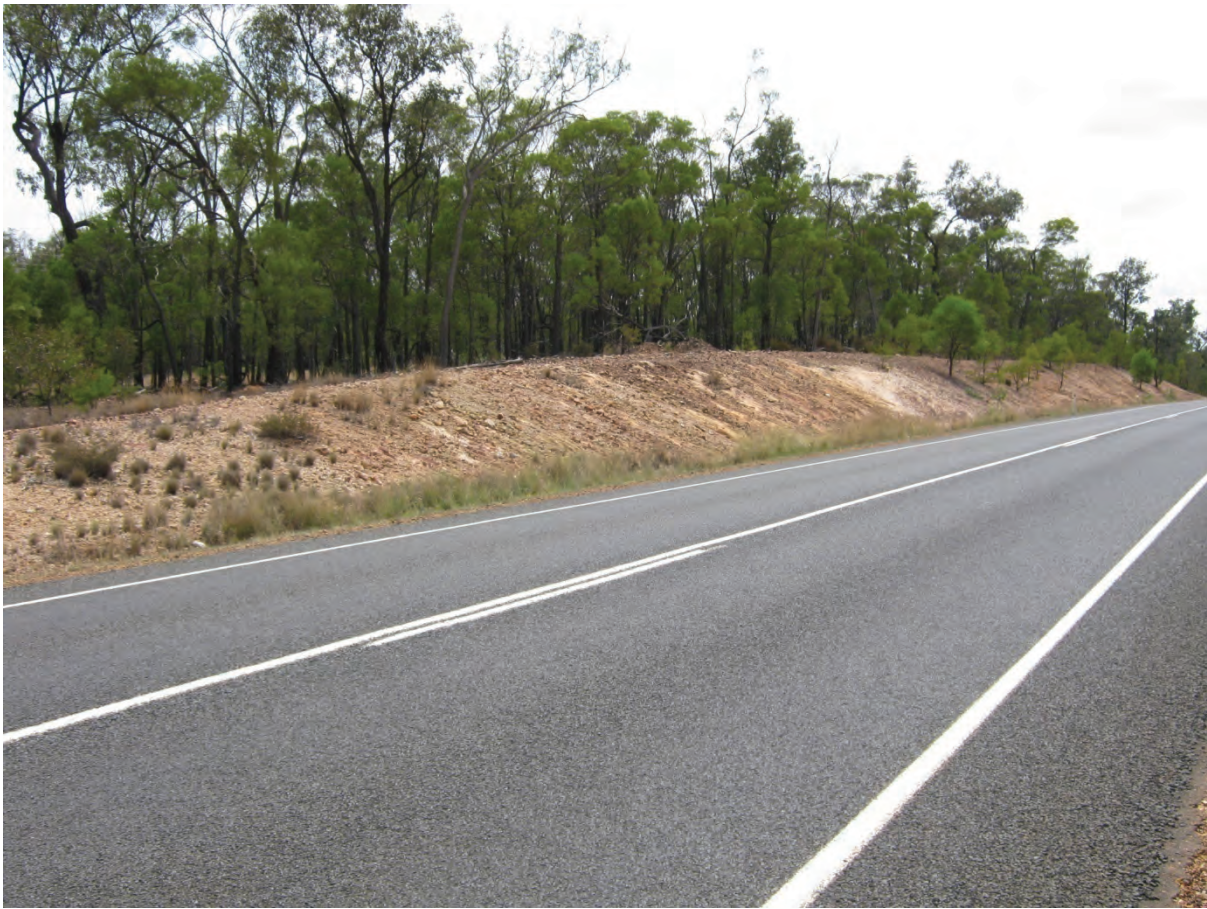
Figure 34: Road cutting, view to Northeast
