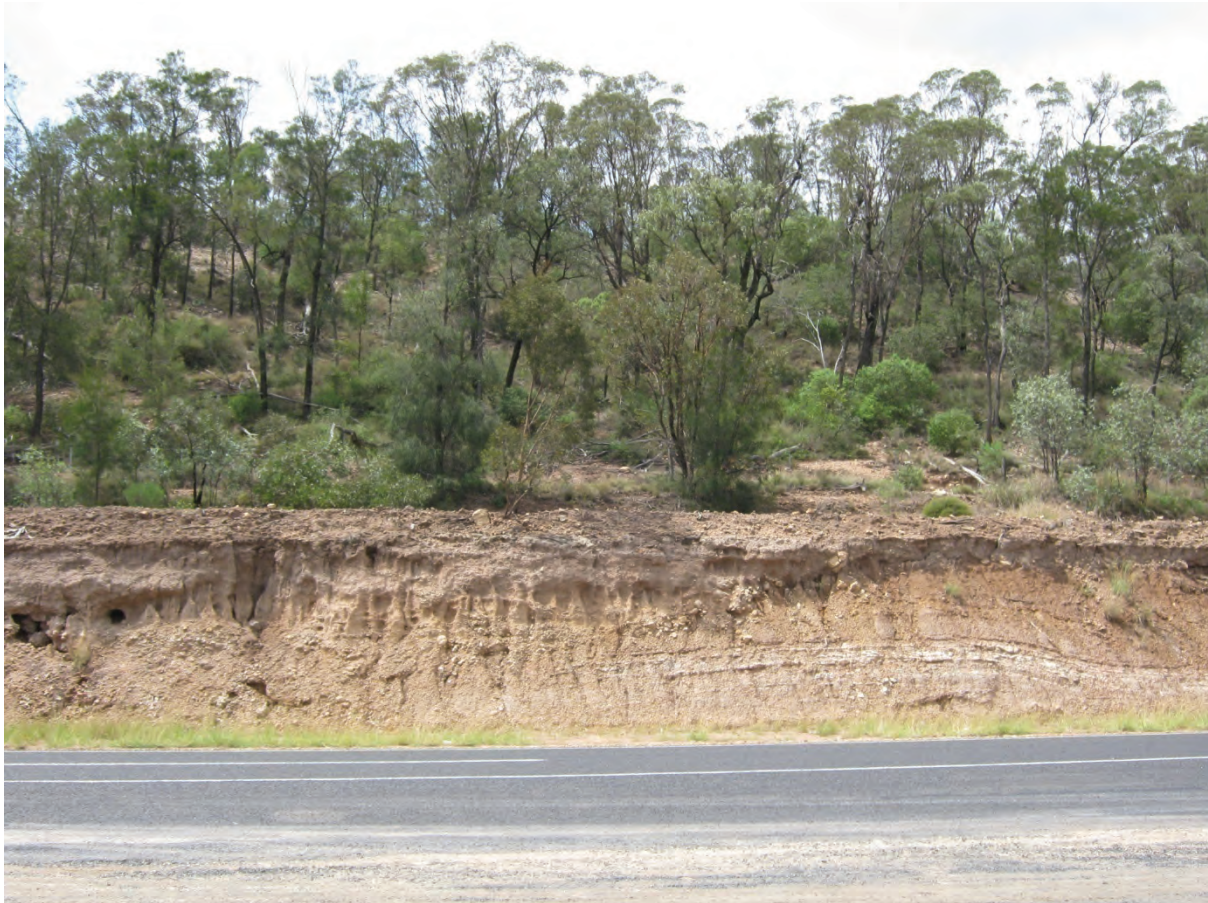
Figure 89: Road cutting, view to Southeast
