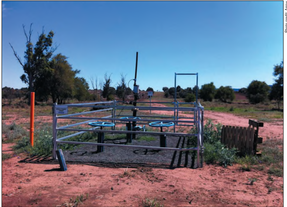
Plate 3.2 Typical surface facility infrastructure for a high-point vent in the water gathering pipeline
