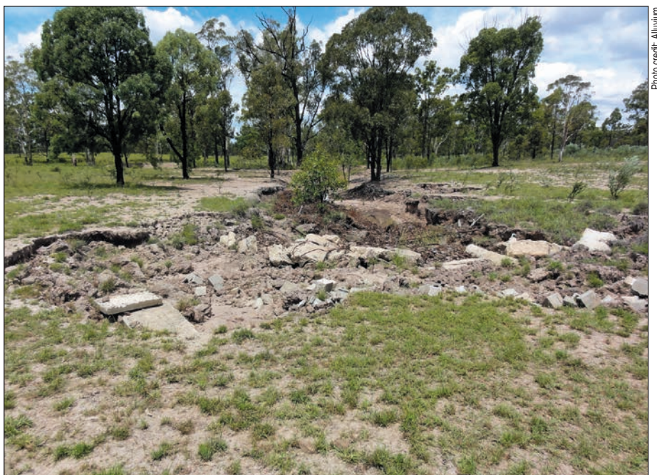
Plate 9.3 Gully showing evidence of headward erosion at the outlet of the farm dam at reach 7 (Bottle Tree Creek tributary)
