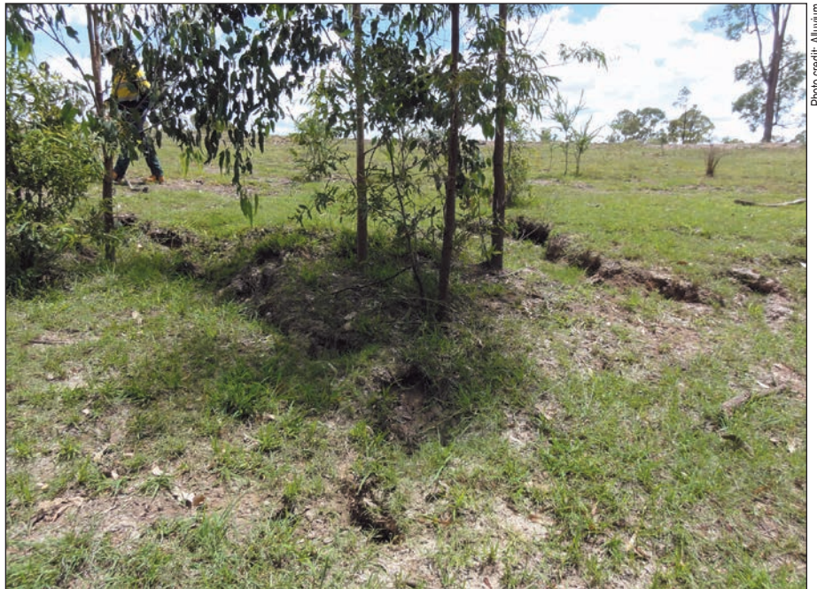
Plate 9.2 Tunnel erosion on the earthen bund built over the original wetland outflow path in reach 5 of Bottle Tree Creek
