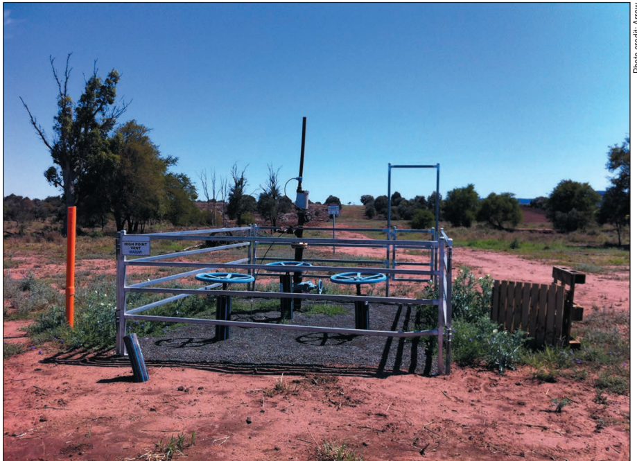
Plate 3.2 Typical surface facility infrastructure for a high-point vent in the water gathering pipeline
