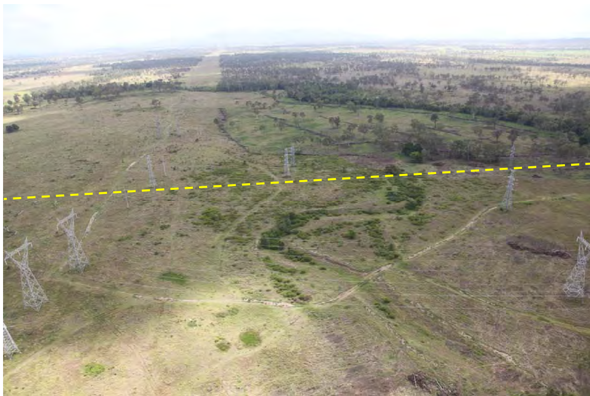
Plate 2.26 View east to proposed pipeline traverse of high voltage transmission line
