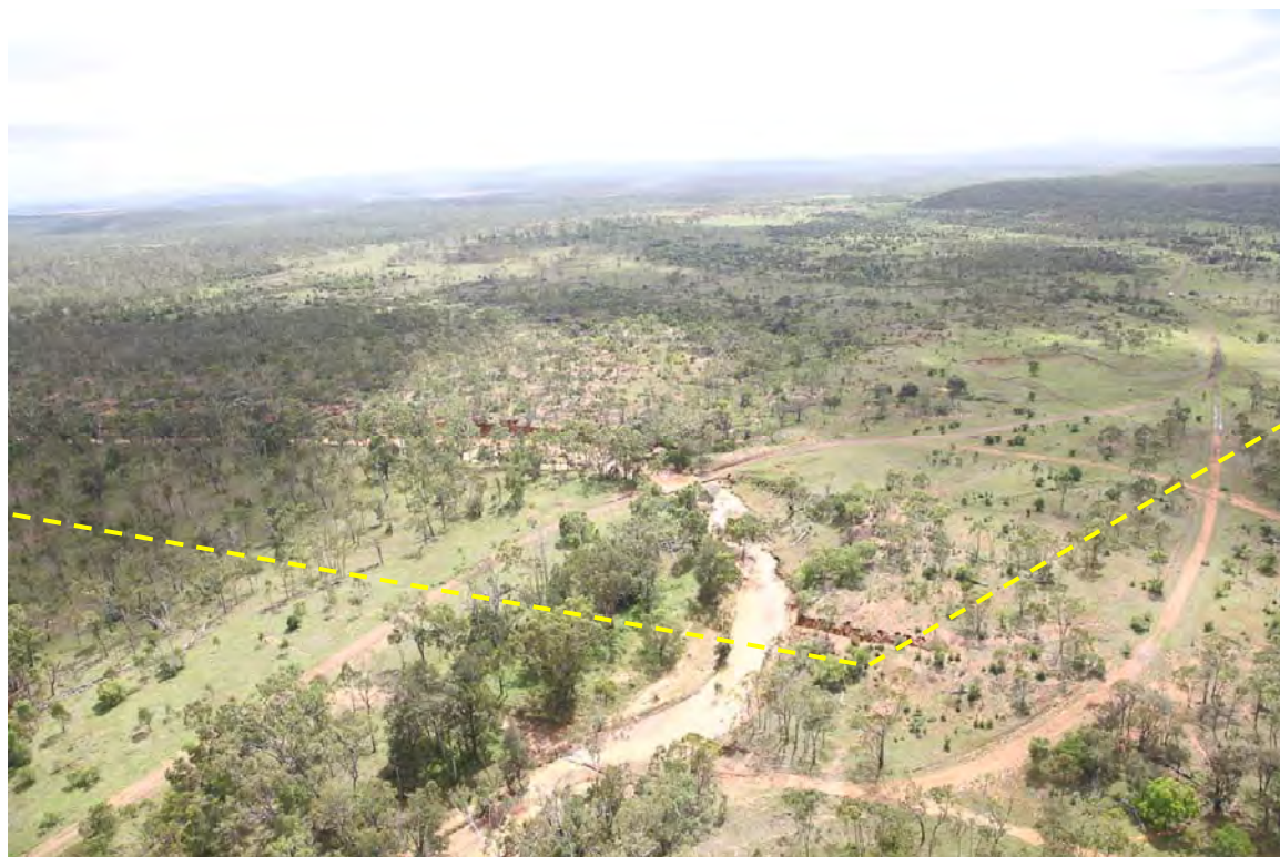
Plate 2.4 View east to proposed pipeline crossing of Teviot Brook (right foreground)
