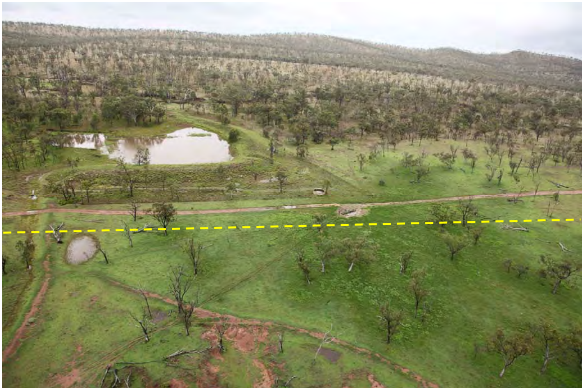
Plate 3.1 View east to dam avoided by the proposed alignment; note gully erosion
