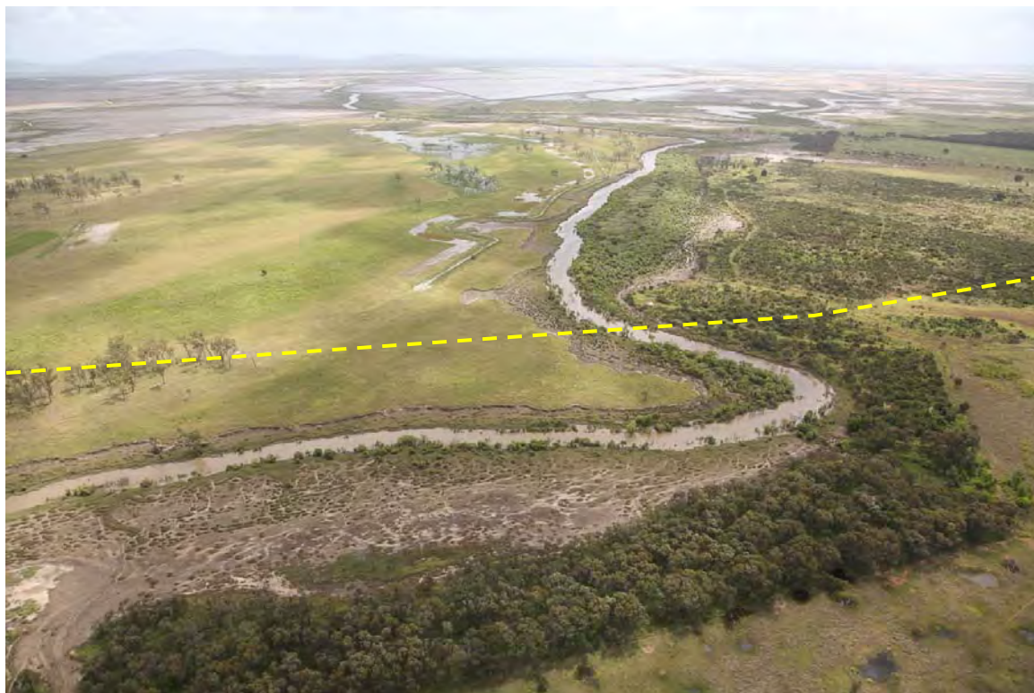
Plate 2.28 View northeast to crossing of Eight Mile Creek; creek tidal at this point
