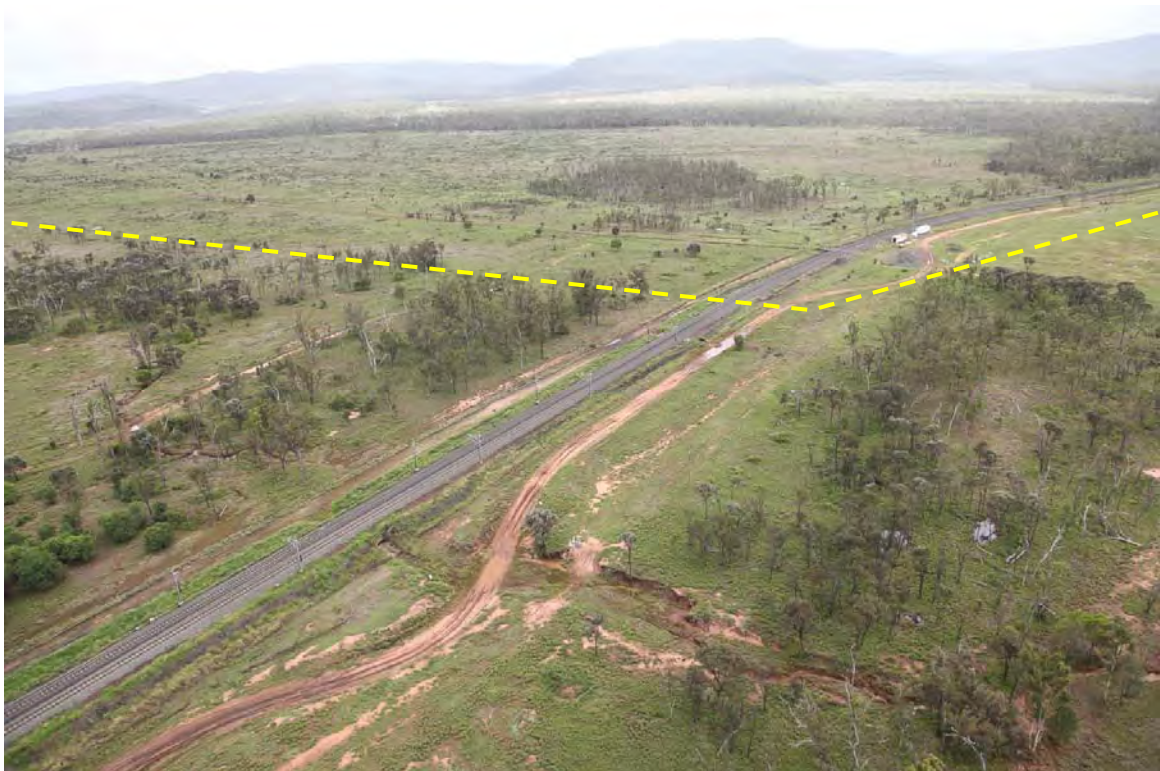
Plate 2.7 View northeast to proposed pipeline crossing of Goonyella Branch Railway
