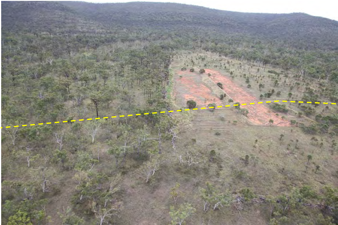
Plate 3.2 View northwest to possible future borrow pit showing topsoil stripping
