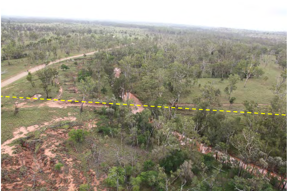
Plate 2.10 View south to proposed pipeline crossing of North Creek at existing track
