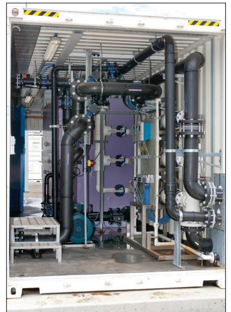
Plate 5.2 Water treatment facility (reverse osmosis plant)
