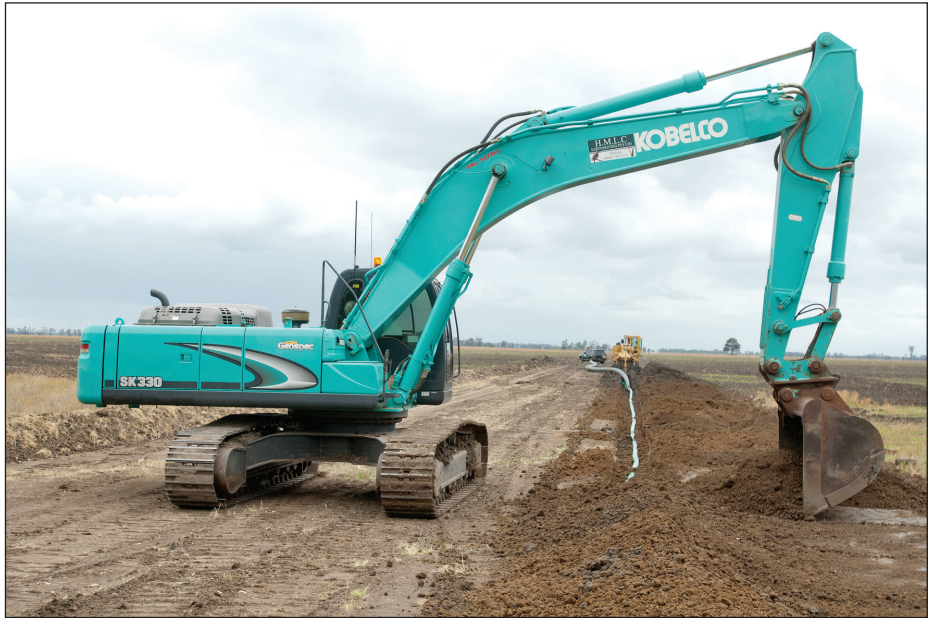
Plate 5.7 Backfilling trench
