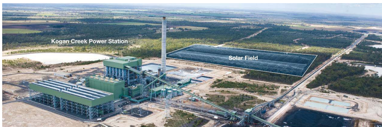
Figure 44 An aerial impression of where the Solar Boost Project will be constructed at Kogan Creek Power Station (source: CS Energy (2011) Kogan Creek Solar Boost Project , (URL: http://www.csenergy.com.au/userfiles/file/Kogan%20Creek%20Solar%20Boost%20fact%20sheet%20April%202011.pdf )
