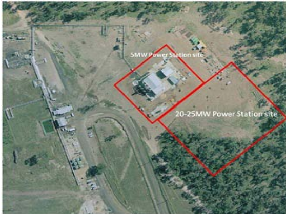
Figure 43 Location of the Proposed Stage 2 Bloodwood Creek 25MW Power Station site (source: Carbon Energy (2008) Bloodwood Creek Queensland Phase 2 Power Generation , (URL: http://www.carbonenergy.com.au/index.php/projects/bloodwood-creek-queensland )
