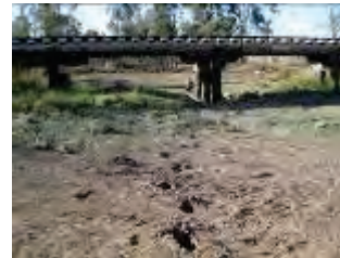
081 – 11 upstream of bridge
