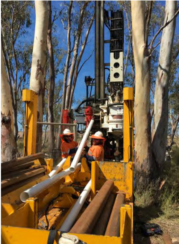
Figure 15. Construction of groundwater monitoring bore at Long Swamp 35.
