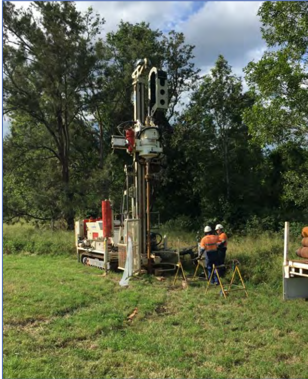
Figure 11. Commachio MC900 sonic drilling rig in the field.
