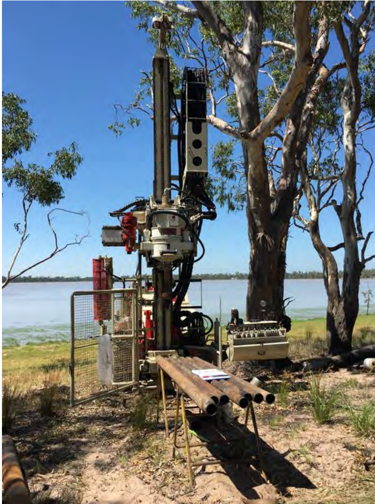
Figure 12. Commachio MC900 Sonic Drilling Rig operating at the Lake Broadwater Study Site.
