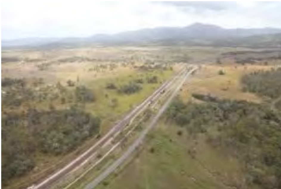
Plate 3-18: View east to crossing of Gladstone-Mount Larcom Road and North Coast Railway
