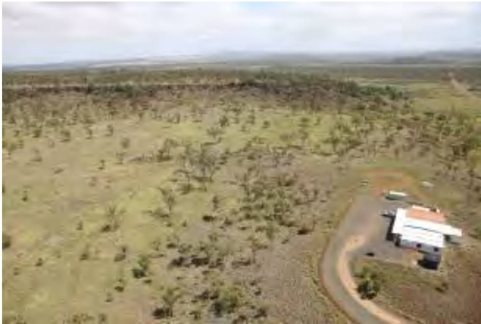
Plate 3-4: Proposed pipeline route lies between ridge to north and the Vale ML to the bottom of the photo
