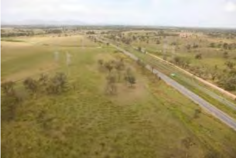
Plate 3-15: View southeast to crossing of Capricorn Highway and Central Railway
