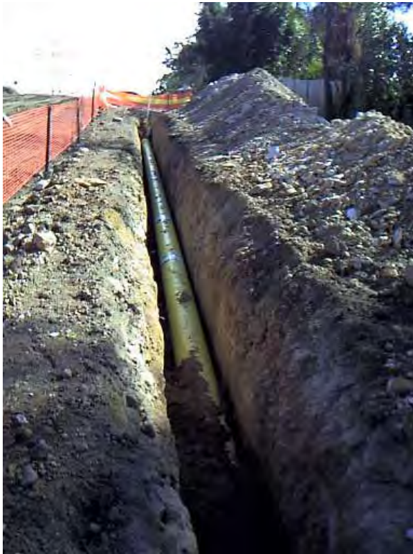
Plate 3-33: Pipe lowered into trench before backfilling
