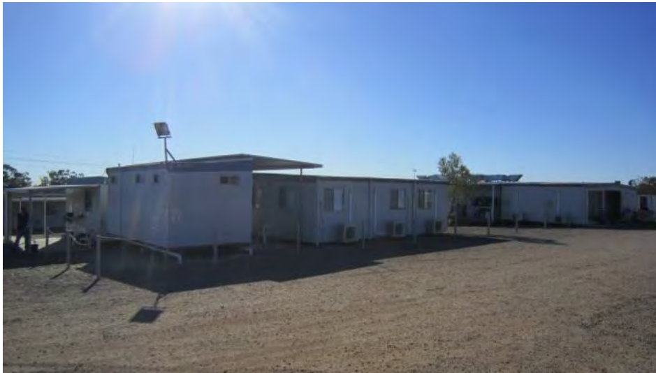
Plate 3-48: Typical temporary workers' accommodation camp
