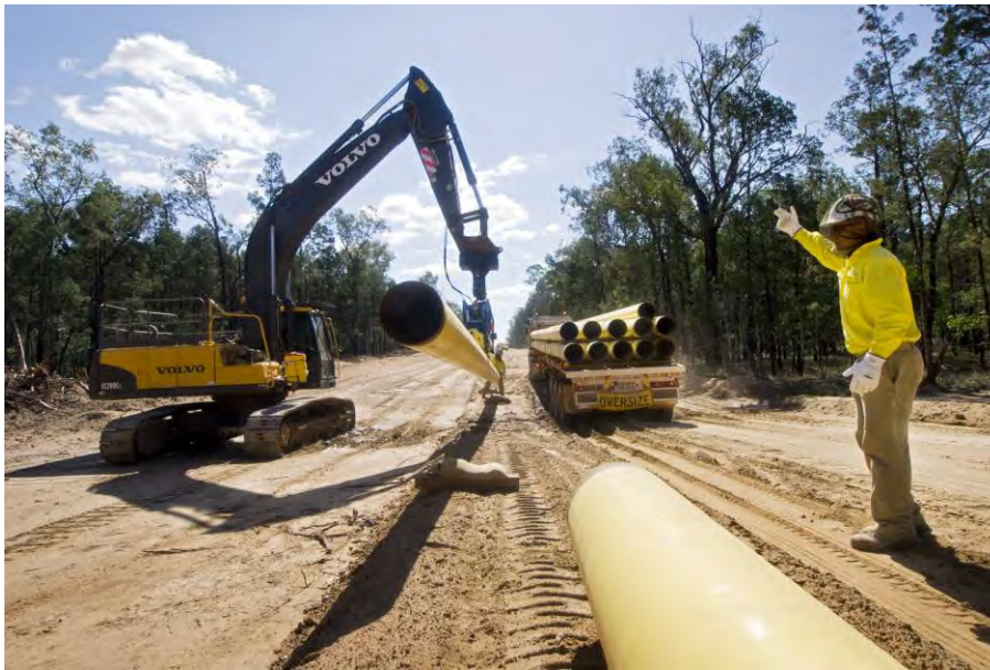
Plate 3-25: Pipeline stringing
