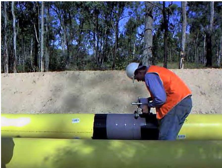
Plate 3-28: Coating of the weld point
