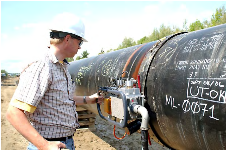
Plate 3-27: Non-destructive testing being conducted
