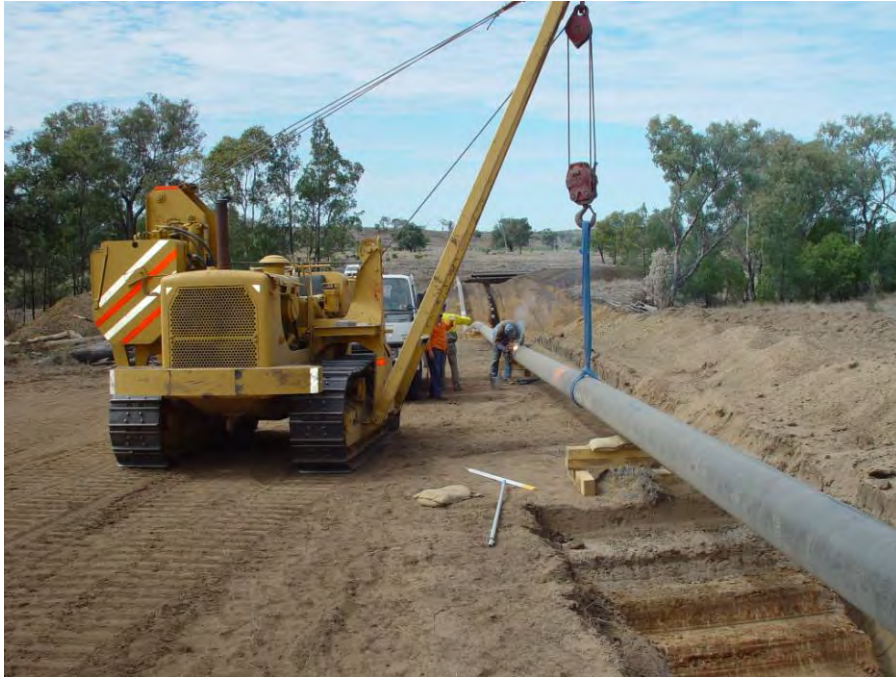
Plate 3-31: Pipe after welding and coating before lowering-in
