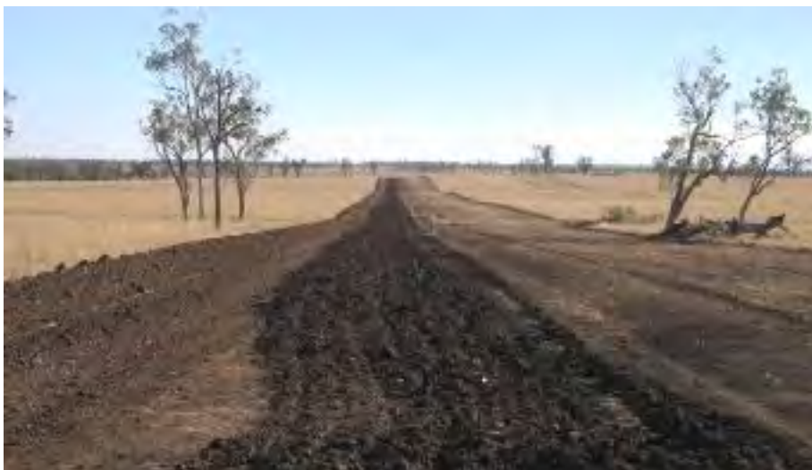
Plate 3-53: Clean up of ROW
