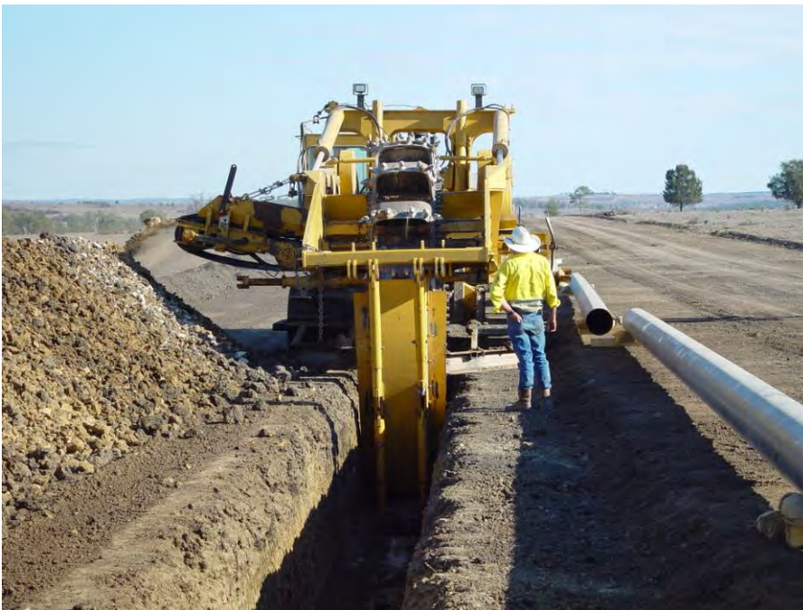
Plate 3-29: Trenching machine in operation
