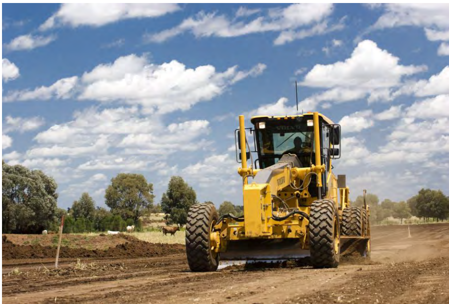
Plate 3-23: Typical grading of the ROW
