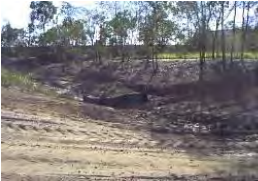
Plate 3-37: Open cut construction of watercourse crossing
