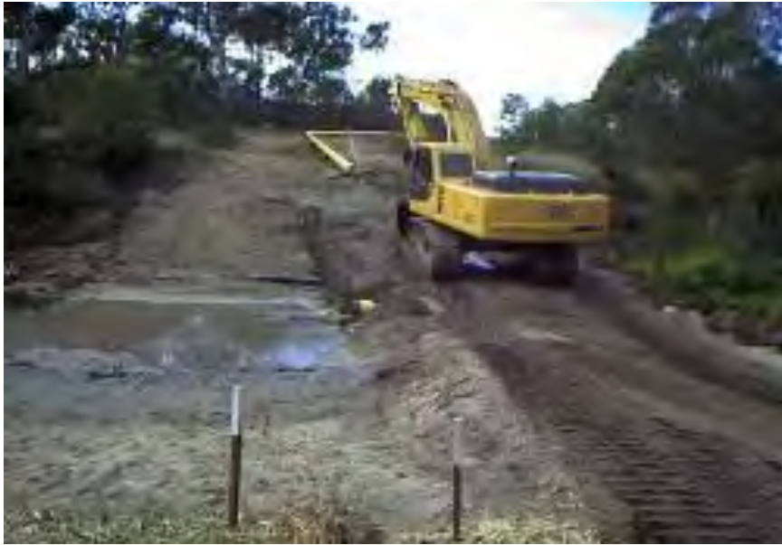
Plate 3-39: Open cut construction of watercourse crossing
