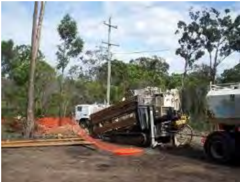
Plate 3-44: Horizontal directional drilling under a watercourse
