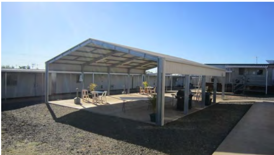
Plate 3-49: Typical temporary workers' accommodation camp
