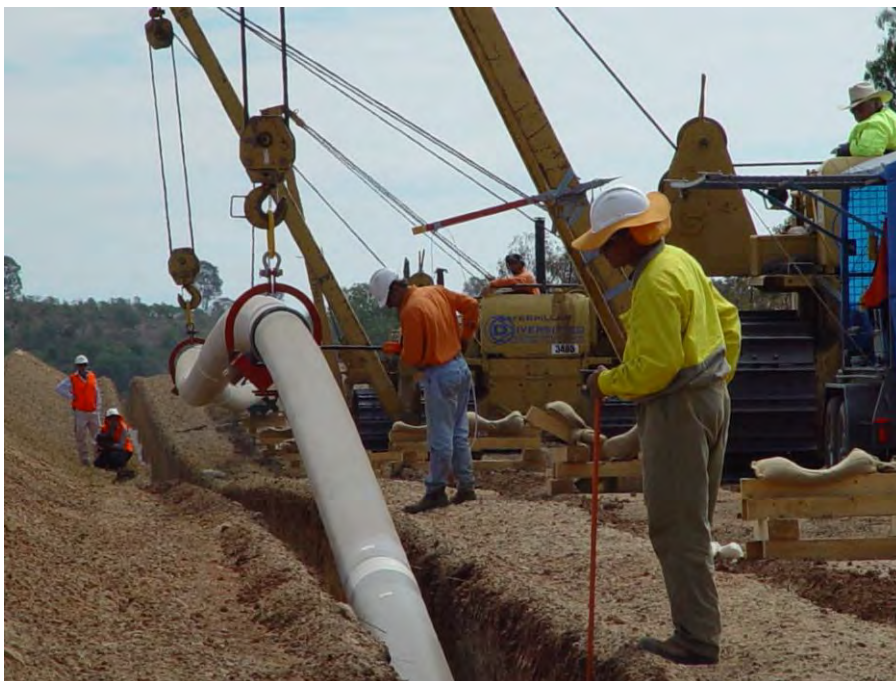
Plate 3-32: Pipe being lowered into trench
