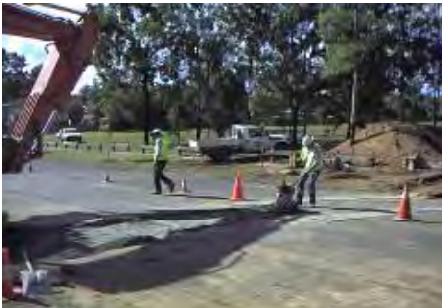
Plate 3-54: Rehabilitation of ROW across a road
