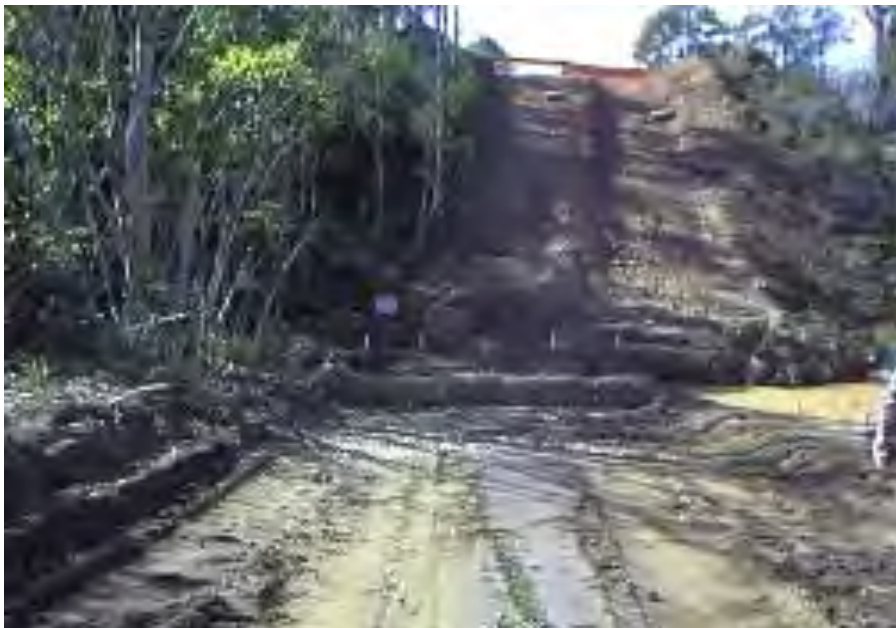
Plate 3-38: Open cut construction of watercourse crossing
