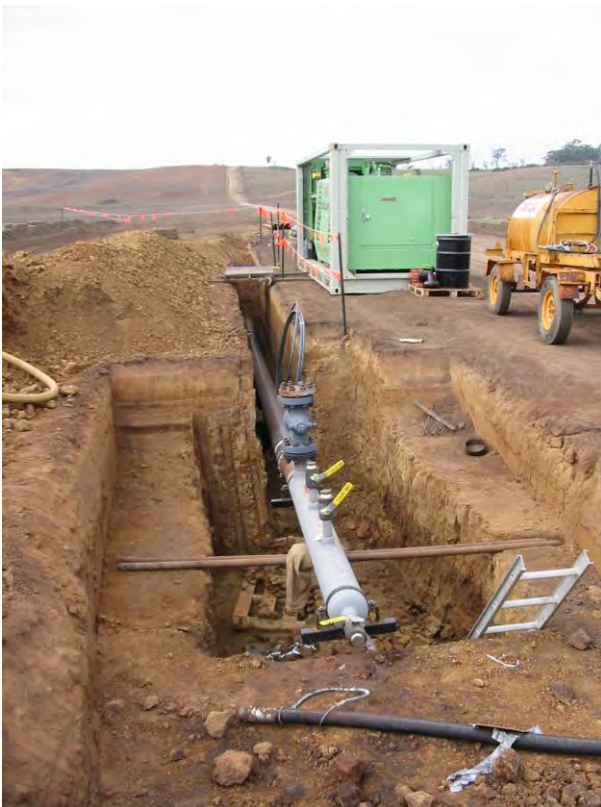
Plate 3-35: Hydrostatic testing in progress
