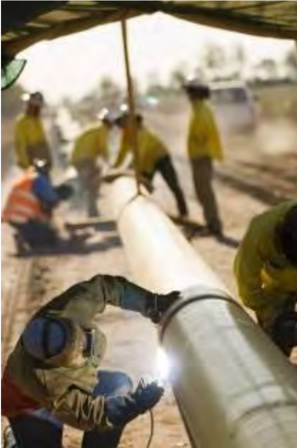
Plate 3-26: Pipeline welding
