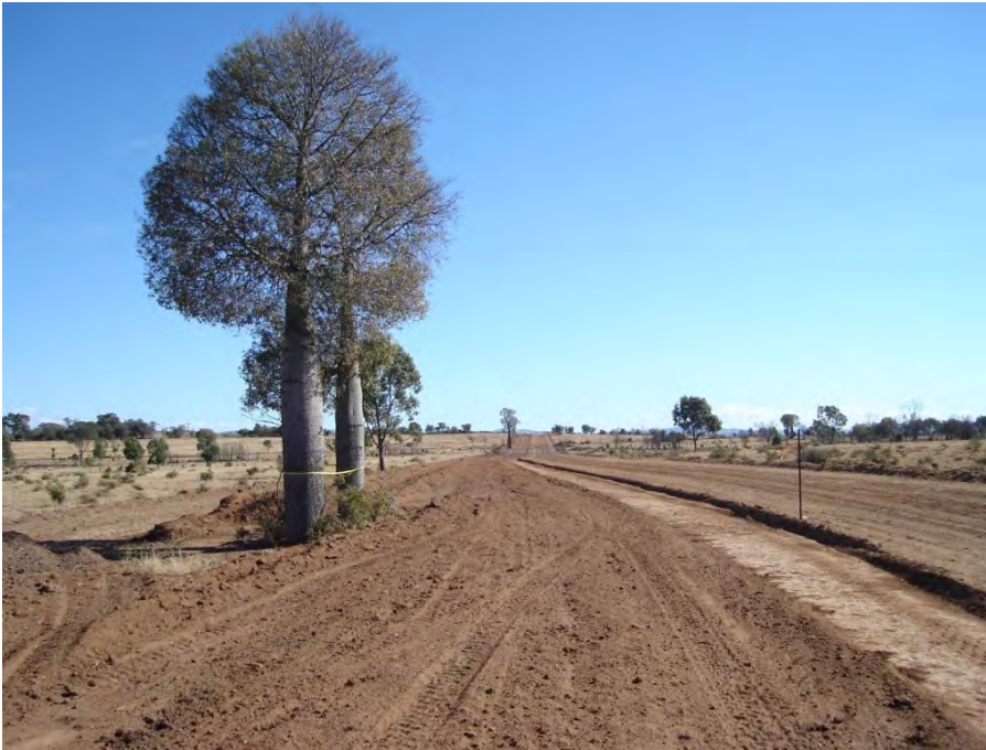
Plate 3-24: Typical clearing of the ROW and avoidance of sensitive vegetation
