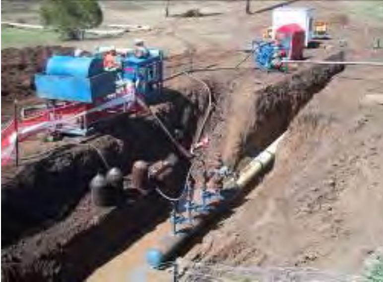
Plate 3-34: Hydrostatic testing in progress
