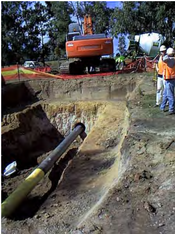
Plate 3-51: Thrust bore under road
