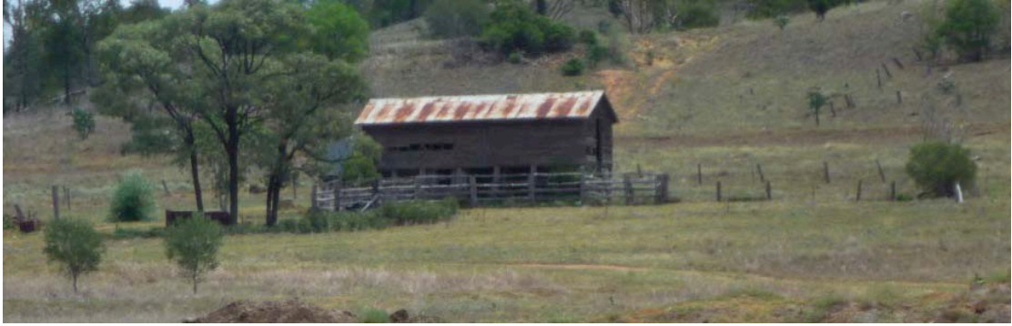
Large barn/ dairy west of Captains Mountain Road. The second school and later the hall were adjacent to the barn.
