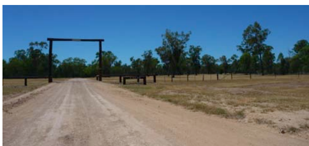
Entrance to Kindon Station.
