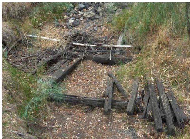
Remains of earlier bridge. below to the south. Railway bridge beyond.
