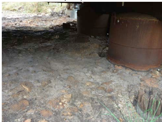
Remains of earliest wooden bridge posts embedded in current bridge footings.
