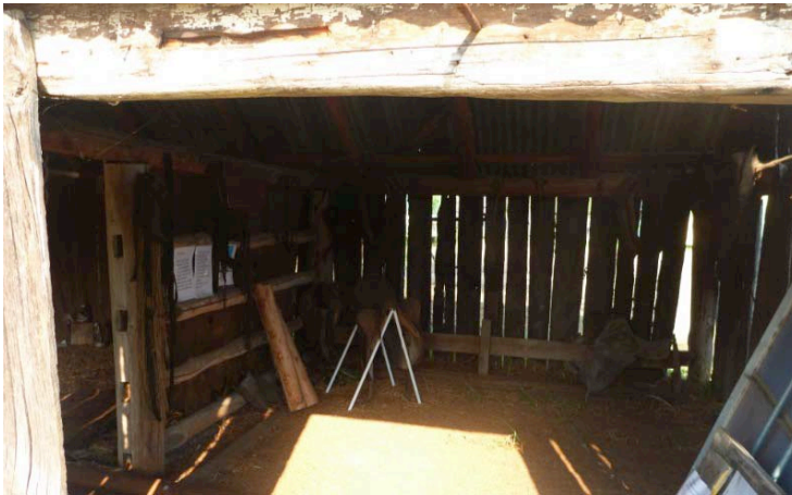
Henry Stuart Russell founded Cecil Plains Station in November 1841. The stables were built c1842. Constructed with adzed timber, hand drawn nails, split timber roof shingles.
