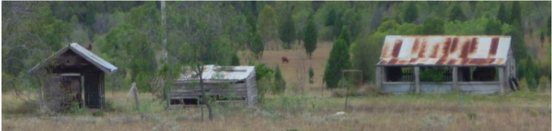
Farm buildings east of Captains Mountain Road.
