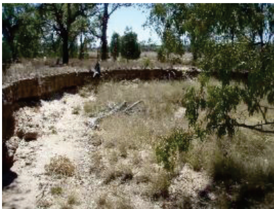
Minor watercourse – laterally active, cut bank erosion. E 314075 N 6957026
