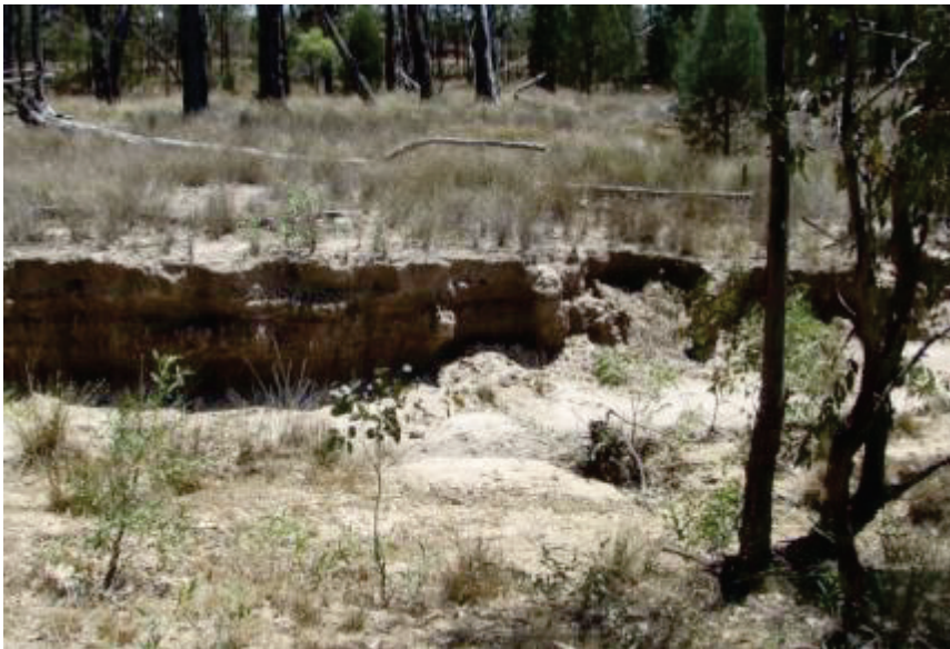
Figure A5-10. Example of active bank erosion following incision of a chain of ponds
