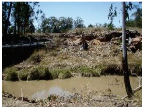
Impingement on indurated Tertiary sediments controlling lateral movement
